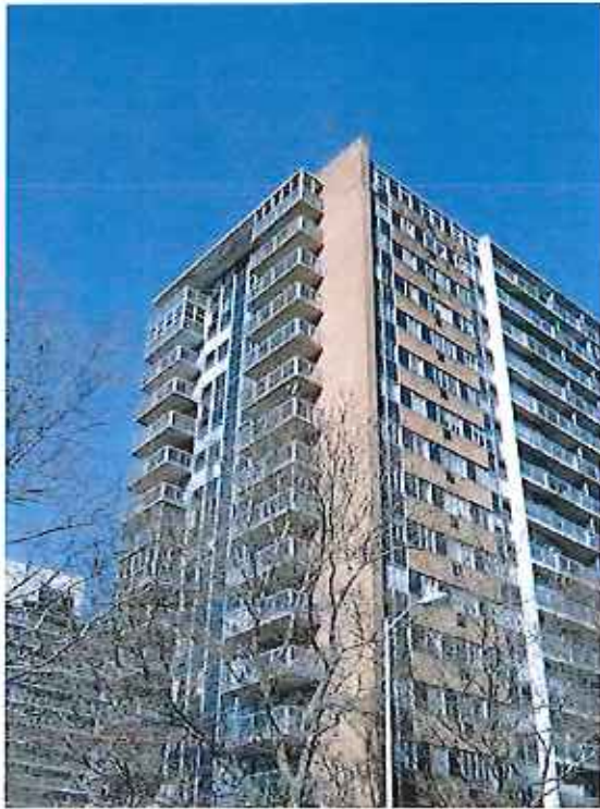
University Towers Owners Corporation New Haven, CT
